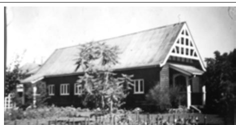
Chapel showing new porch on western end
